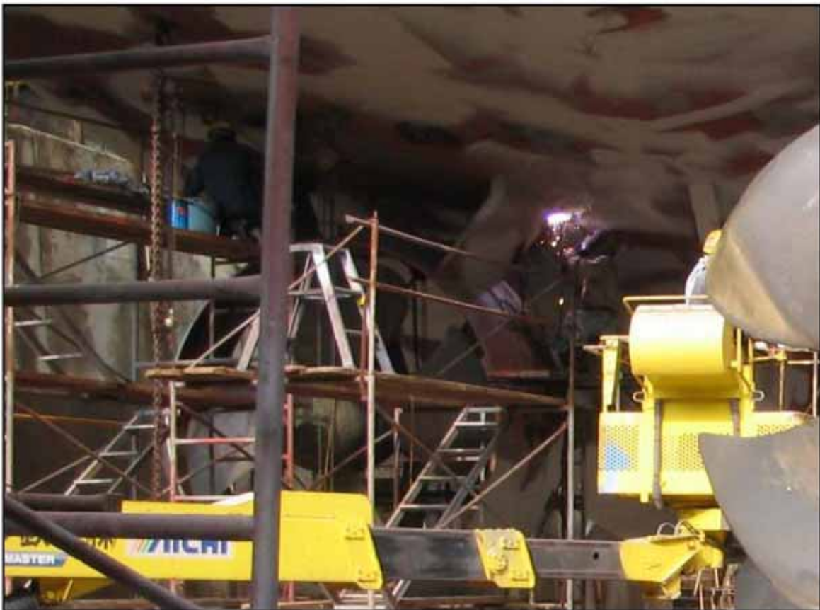
Figure 28: Photograph of worker repairing the inboard port Kort nozzle strut
